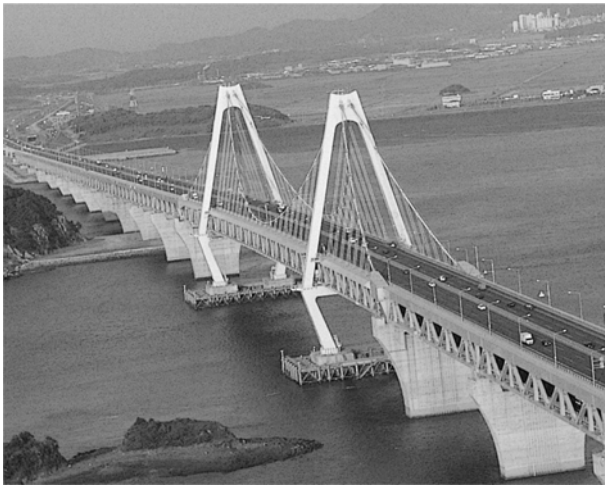
Figure 7. Yongjong suspension bridge.
