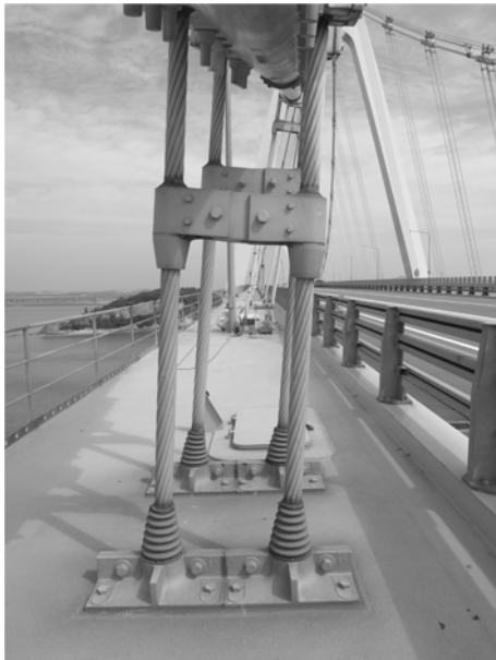
Figure 8. Double hanger system (NTS03).
